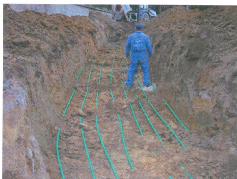
Fig 6 . A horizontal heat exchanger is being mounted in Barcelos (Portugal) [9].
