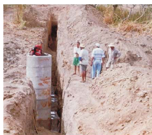
Fig. 10 - Ditch Pit Excavated and Amazon Source: {14}.
