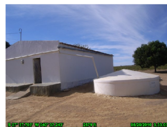
Fig. 8 - Tank plate to capture rainwater that runs off the roof of the house.
